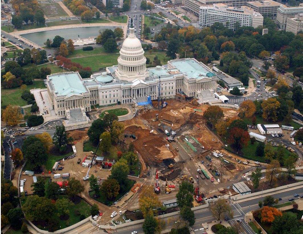
Construction of the Capitol Visitor Center in 2006
