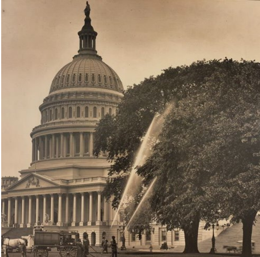
101 Chemical application operation, circa 1910.
